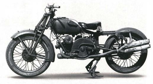
A 1945 picture of the 'Alce,' with the outside flywheel clearly in evidence.
